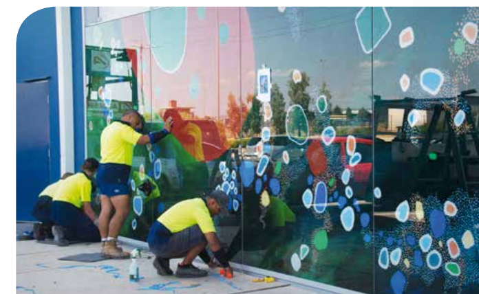
Cooling Brothers Glaziers installing the double glazed units
